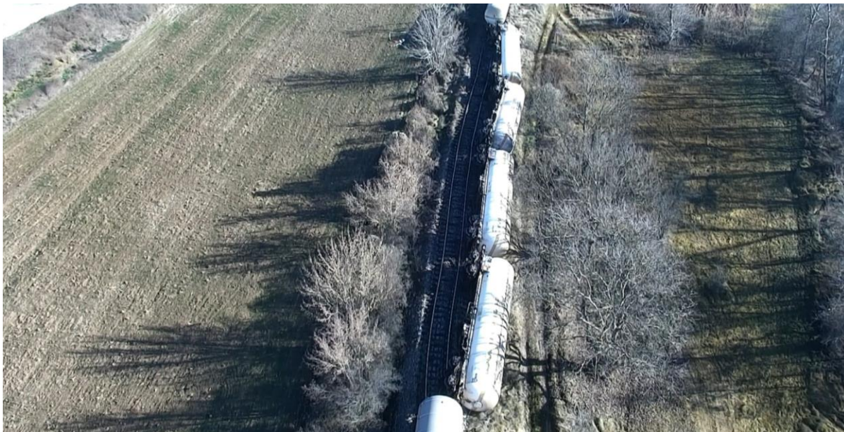
Figure 4.1.1.2: Appearance of the point of overturning of the wagons-tanks (source: MUP, Emergency Situations Sector)
