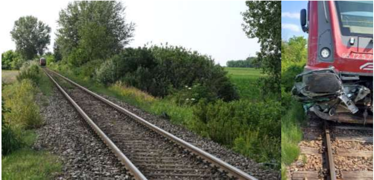
Figure 3.3.2: View of the stopping location and Train No. 25442
