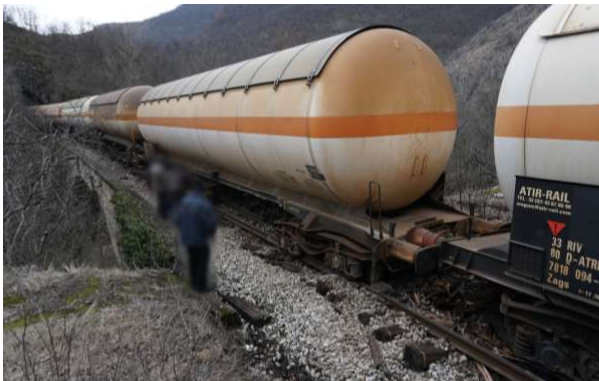
Figure 4.1.1.1: Review of the derailment point (concrete bridge between Tunnel No. 21 and Tunnel No. 22)
