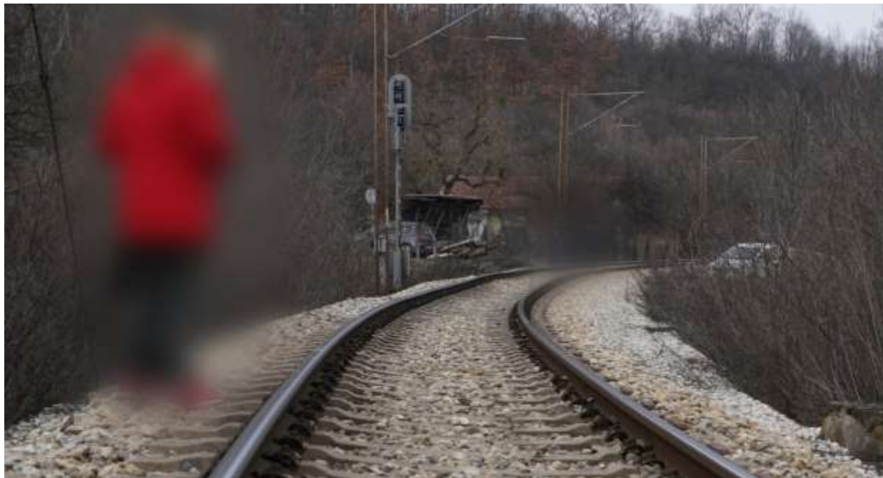
Fig. 3.1.1: View of the derailment site (looking in the direction of train travel)
