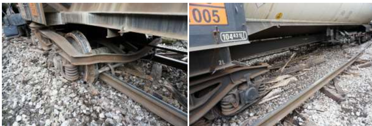
Figure 4.1.1.2: Review of the parts of the derailed wagons
